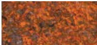
Without corrosion protection treatment
